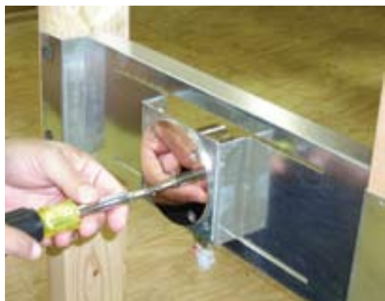
SolidDrive SD1 drywall installation during new construction View from behind
